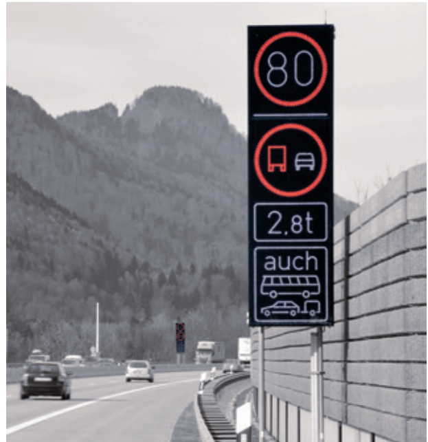
06 LED variable message sign (LED VMS)
