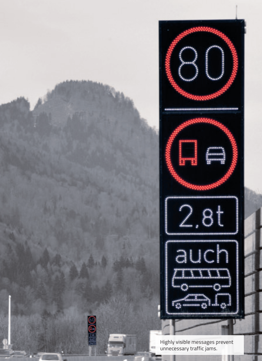
The front panel is made of printed polycarbonate.
